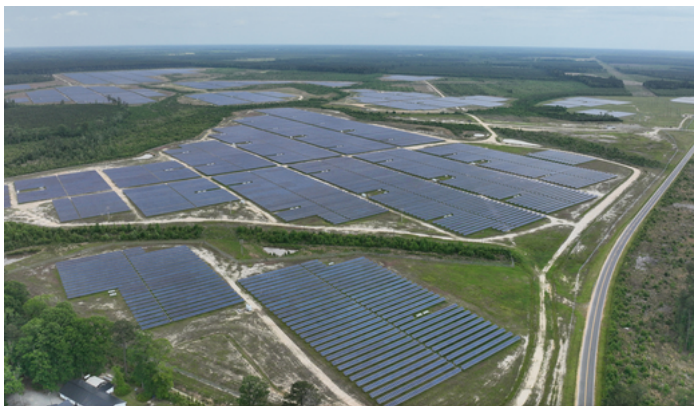
The Aulander Holloman solar project in North Carolina.
